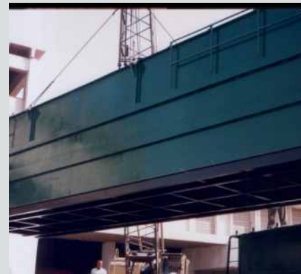
Crude Oil Storage Tank
