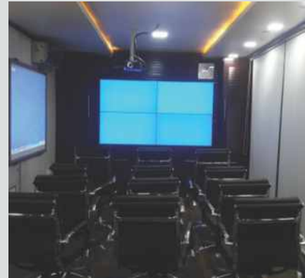
Command & Control Trailer (Inside view)
